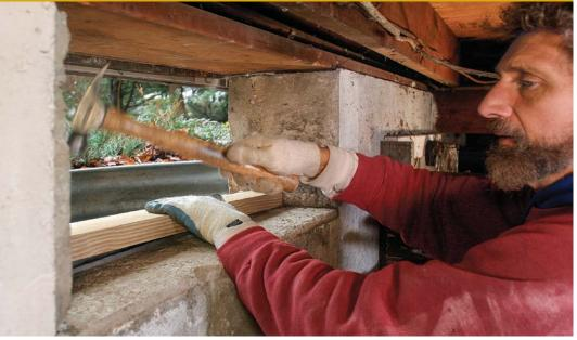
Fit the sill. Cut correctly, the sill should fit snugly, requiring a few taps of the hammer to seat it in position. To attach the sill, drill and drive concrete screws into the concrete below.
