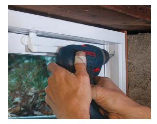
Into the bucks. Screw through the sides of the window and into the side buck pieces. Use screws that are long enough to bite into the wood but not so long that they bottom out on the concrete beyond.
