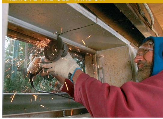
Split the window down the middle. After removing the window sash, use an angle grinder with an abrasive cut-off wheel to make two front-to-back cuts through the metal frame: one across the top and one across the bottom.
