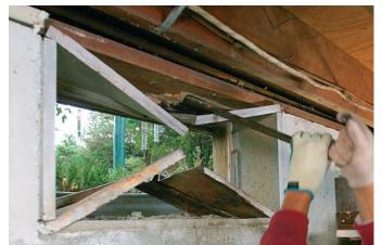
Pry the old frame out. Use a pry bar to bend the top and bottom of the frame toward the center, allowing the sides to be pulled inward. After prying the top of the frame down in the middle, use a reciprocating saw to cut the outermost portion of the top flange. This is done usually from the exterior side of the window.
