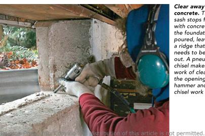
Clear away excess concrete. The hollow sash stops filled with concrete when the foundation was poured, leaving a ridge that now needs to be chiseled out. A pneumatic chisel makes quick work of cleaning up the opening, but a hammer and masonry chisel work fine, too.
