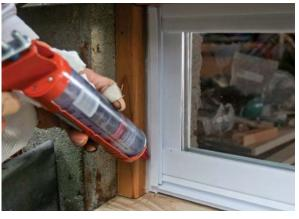
**Extra insurance.** Finish the job with a bead of sealant around the interior and exterior perimeter of the window frame, except along the exterior at the sill, which is left open for drainage.
