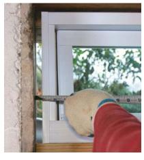
Measure the opening. With the window resting in place on the sill and centered in the opening, measure the width of the gaps at several points of each vertical side to determine if the bucks need to be tapered.
