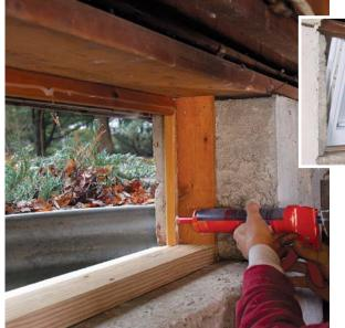
Install the window. After applying sealant to the inside face of the window stops, slide the window into the opening. If the window fits a little too snugly between bucks, don't force it into place and risk damaging it. Use a block plane to shave down the side channel of the vinyl frame.
