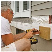
Gauge blocks guide the ledger. After determining where the ledger will attach in relation to the benchmark line, mark the offset on both ends of a pair of 2x8 cutoffs—the material that will be used to frame the landing. Align the marks on the blocks to the benchmark line, and screw them to the wall.
