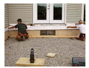
Any level line will do. You don't have to bother adjusting the height of a laser to project a ledger guideline at just the right elevation. Instead, project a level line somewhere near where the ledger will attach, and then snap a line to be used as an offset benchmark for the rest of the elevations.
