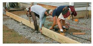
**Align and fasten.** One person holds the two halves of the beam so that the tops are in alignment before the second person nails them together. Building codes recommend the use of 10d threaded nails set in two staggered rows, with 16 in. between nails. The author nails more liberally.
