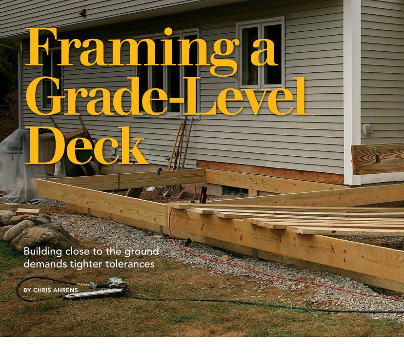
he traditional raised deck frame is a beautiful balance of structural function and adjustability. A ledger attaches through the wall sheathing and into the floor frame of the house, joists extend out from the ledger across the top of a built-up beam, and weight is transferred down support posts to footings below. The height of the deck is usually driven by the elevation of the house's floor framing, and then a set of stairs runs from the deck to the ground.
