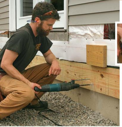
**Nuts before hammers.** Use the predrilled ledger as a template for boring the holes in the concrete. But before whacking the wedge anchors into place, put a washer and a nut onto each bolt. A hammer can damage a bolt's leading
