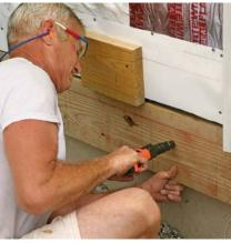
Two nails let you focus on the drilling. Lift the ledger so that it's tight against the bottom edge of the gauge blocks, and then shoot a powder-actuated nail into each end of the ledger to tack it in place. Drill a hole and set a bolt on each end of the ledger before drilling all of the other bolt holes.
