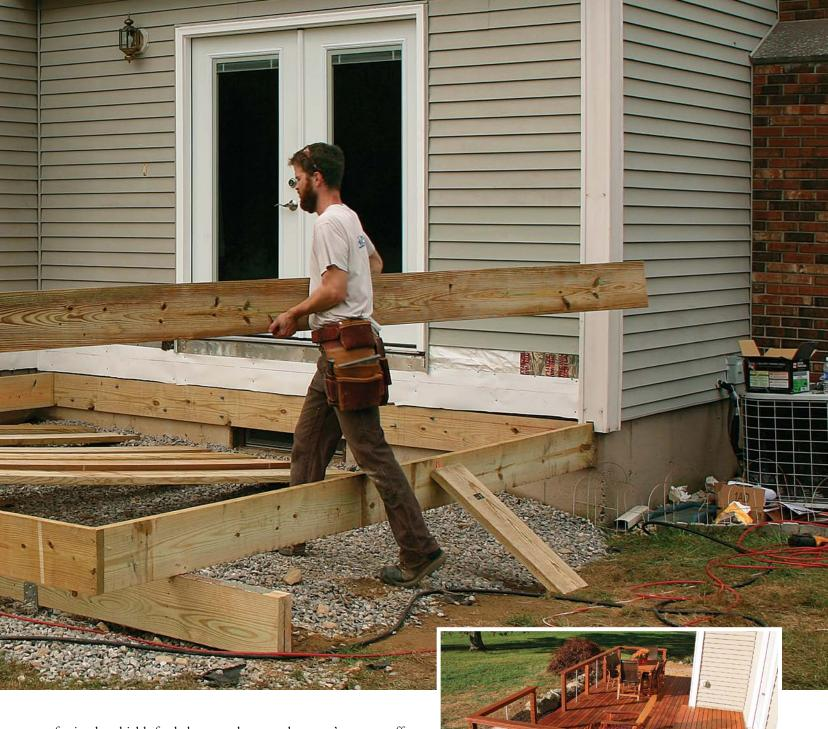
of using lag shields for ledger attachments; they aren't up to snuff for structural deck connections. You can't use wedge bolts if you're attaching to a hollow-block foundation, but adhesive anchors will do the job as long as you set them in mesh screening or tubes, which gives the adhesive solid purchase inside the hollow block.
