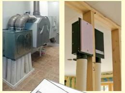
Distribution breakdown The 10 corrugated ducts bringing stale air to the ERV must be balanced by the 10 ducts supplying clean air from the ERV. Each duct is designed to carry 12 cfm. Here's how the distribution works in this house.
