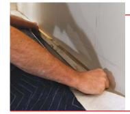
You don't need to screw in a ledger behind the oven to support the first row of tile. Instead, cut a piece of wood so it can be pressure-fit between the countertops.
