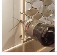
Screws driven into drywall offer enough holding power to temporarily support tiles that are sliding out of alignment.
