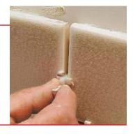
with the field tile, not worrying about any grout that oozes into the area of the mosaic accent. Once the grout firms up somewhat, it's easy to clean out the joints with a utility knife. Then when I'm ready to grout the mosaic section, the surrounding field-tile grout will have firmed up enough so that I can wipe away any overgrouting with a sponge.
