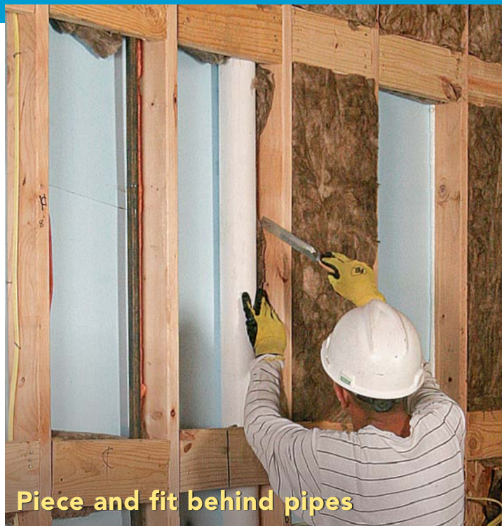
Fill around refrigeration lines
