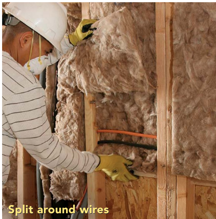
Use scraps when necessary
