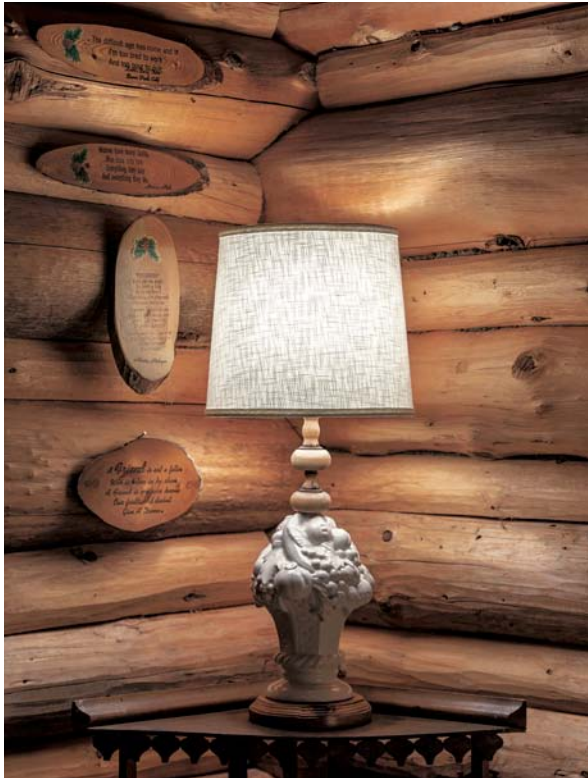
Corner weave. Alternating logs of smaller and larger diameter are critical to the stability of the walls of a log house. This effect is best seen at the corners. Here the logs are shown from the interior (above), as well as the outside (below), where the dark log color comes from the use of creosote as an early wood preservative.
