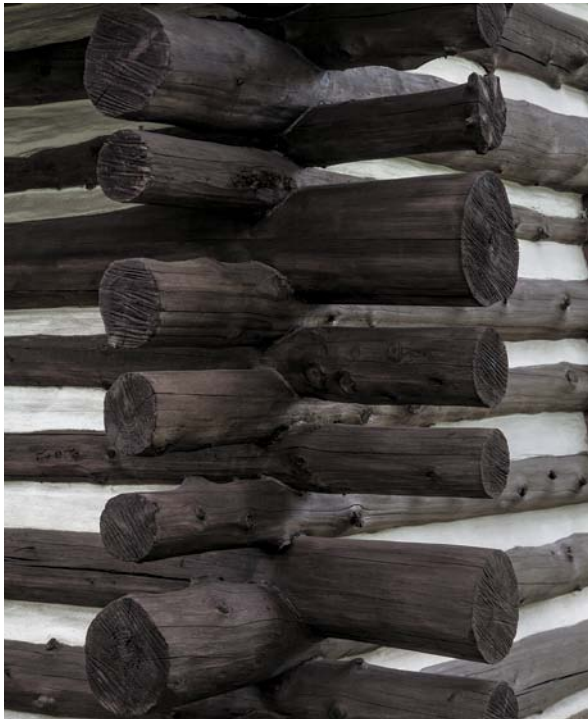
Corner weave. Alternating logs of smaller and larger diameter are critical to the stability of the walls of a log house. This effect is best seen at the corners. Here the logs are shown from the interior (above), as well as the outside (below), where the dark log color comes from the use of creosote as an early wood preservative.
