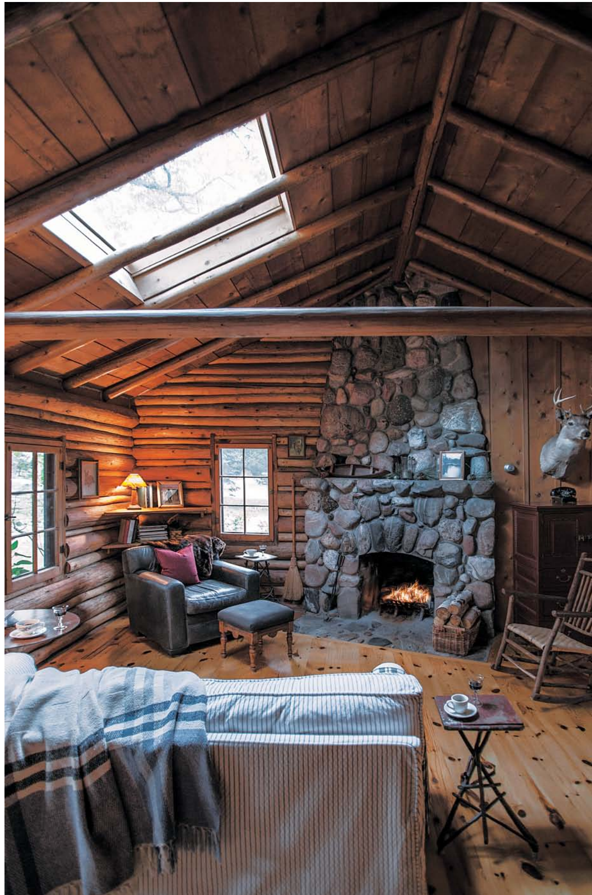
Lightening up. Skylights were added to let light into what had been a dark living space.
