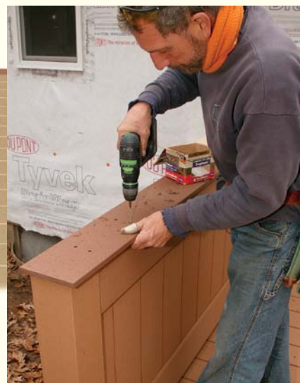
Screw the panel to the posts. Raise the half-clad panel on top of 3-in. spacer blocks, and align it 1/2 in. from the post cover edges. Drive screws through the 2x2s into the posts to secure the panel. Cover the unclad side with black tape, and install vertical trim boards.
