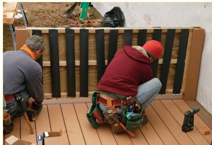
Screw the panel to the posts. Raise the half-clad panel on top of 3-in. spacer blocks, and align it 1/2 in. from the post cover edges. Drive screws through the 2x2s into the posts to secure the panel. Cover the unclad side with black tape, and install vertical trim boards.
