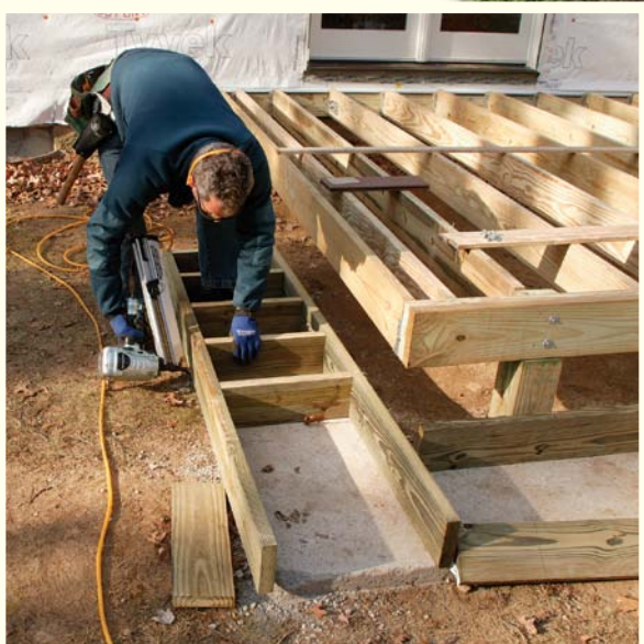
Solid support. The decking manufacturer calls for closer support spacing (12 in. on center) when decking is used for treads. Some manufacturers call for supports to be as close as 8 in. on center.
