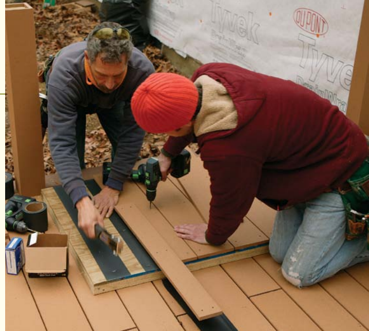
A simple base. Size a 2x2 frame to fit between the two trimmed-out posts, but make it 3 in. shorter than the post height to create a gap at the bottom.
