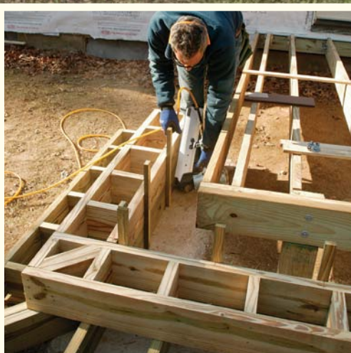
Stack boxes for stability. Build the bottom box frame twice as wide as the top. Diagonal blocking at the corners provides nailing for the mitered treads. This design locks the boxes together so that the outside corner is less likely to open up over time. Tie the boxes together and to the deck frame with 1x straps that match the thickness of the deck skirt, then push the boxes into place.
