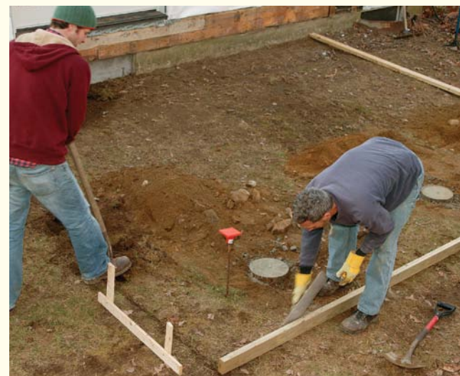
Mark and dig the stair footings. Use a 2x as a straightedge to mark the position of the stair footing pads. Dig square and flat holes to the dimensions of the stair frame. Form the top with 2x stock for even edges at the precise position of the stairs.
