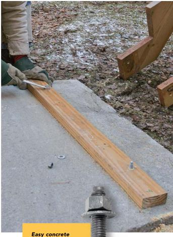
Connector screws don't pull out.
