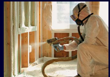
Insulation air barrier. Unlike fibrous insulation, properly installed spray polyurethane provides an excellent air barrier as it fills in around pipes, ducts, and wires and as it seals the gaps between framing and sheathing.
