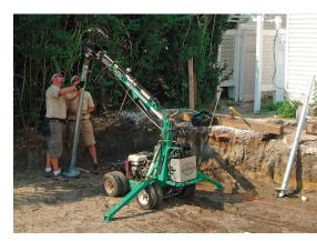
capacity of the footing. Once the required bearing is reached, the pile is cut to length and a beam saddle is welded on. Depending on the contractor, you can end up with an engineer's report that verifies the load each footing can handle. One source for that service is technometalpost.com.
