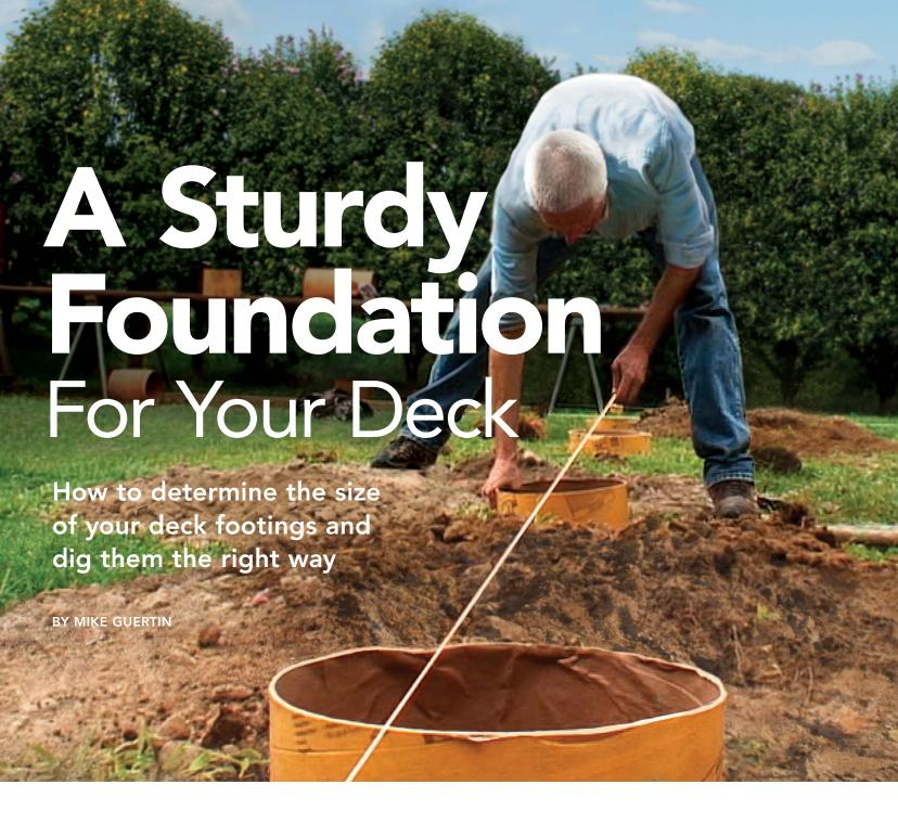
eck footings transfer the weight of a deck and its occupants to the ground, forming a solid foundation to support the deck and its live and dead loads. How many footings you need and how big to make them is specific to each deck. Doing the calculations takes only a few minutes, ensures that I'm following best building practices, and keeps me from digging more than necessary.
