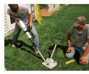
The residential models have a load capacity of 2700 lb. when installed in 1500-psf soil and 3600 lb. in 2000-psf soil. The pins are driven into the earth in just minutes using a 11/8-in. hex-shank demolition hammer.
