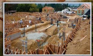
Building on a good foundation. Through integration, general contractor Mike Martuscello and structural engineer Bruce King arrived at a pier-and-grade beam foundation that reduced carbon impacts by an estimated 30 tons and resulted in less environmental impact than that of the lighter mat foundation previously considered.
