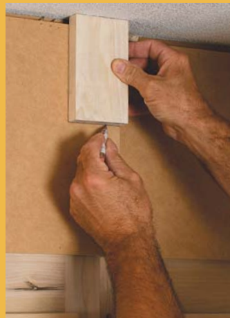
Mark the crown's bottom. Use a block cut to the length of the crown's drop to mark the location of the crown's bottom on the frieze.
