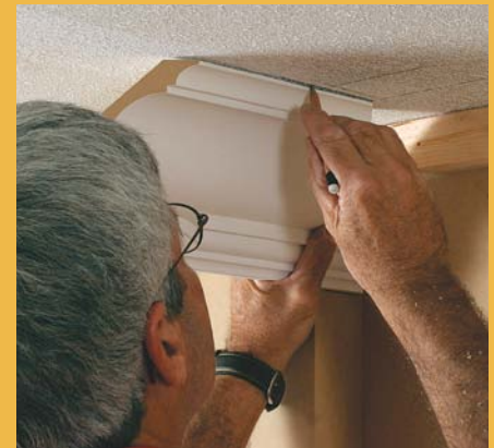
Mark the crown's top. To locate the top, hold a scrap of crown to the bottom line.
