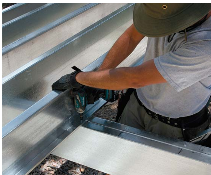
Screw joists to beam. Connect a joist to a beam with a screw between the flanges.
