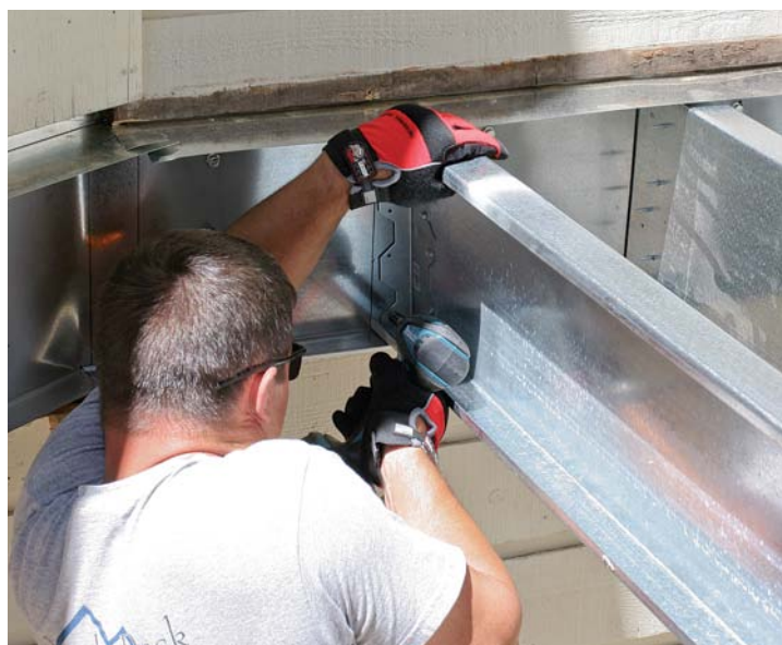
Standard framing angles join joist to ledger. Fasten the framing angle to both members with self-tapping sheet-metal screws.
