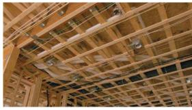
Open-web FLOOR TRUSSES A offer long spans and the ability to run mechanicals between the first and second floors—a saving grace in a house where the attic is off-limits and there is no basement.
