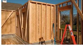
The OUTSIDE FRAME ▲ supports most of the floor load and all of the roof load. It also holds part of the primary air barrier, and with the help of diagonal bracing, provides the necessary windshear resistance for this coastal site.
