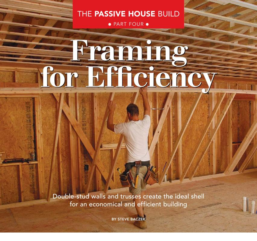
he frame of a Passive House may not be as exciting as the thick layers of insulation, the high-tech mechanical systems, or the tripleglazed windows, but it plays a very important supporting role—pun intended—in achieving success.
