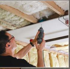
Using a 1/8-in. guided bit in a drywall router, plunge into the penetration, then move over until the bit hits the side of the box, fan, duct, or light.
