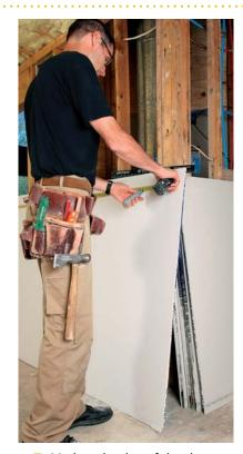
Mark each edge of the sheet. Framing isn't always square and plumb, so if the measurements differ, use the shorter one. There's no need for a pencil; mark the cut with a knife tick.
