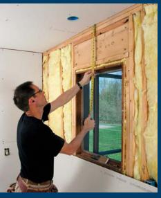
Measure the distance from the ceiling to the top of the opening, and from the opening's edges to the nearest wall or installed sheet of drywall. Mark these measurements in the face of the board.
