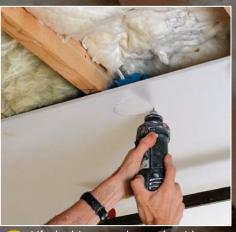
Lift the bit out and over the side of the penetration, then reinsert it. Keeping the bit in contact with the outside surface of the penetration, move the router in a counterclockwise direction.
