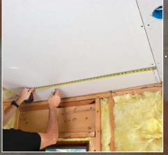
If the penetration is in the middle of a board, note its distance from adjacent walls or already-hung sheets of drywall. Hang the board, then mark the center of the penetration on the face.
