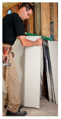
Once scored, place one hand on each side of the cut, gently lift, and bend the board backward to snap the gypsum core.
