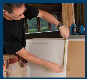
To cut the long edge of a drywall sheet, pinch a tape measure at the desired measurement, then slide your fingers along the edge of the drywall while holding the knife against the hook at the other end of the tape.
