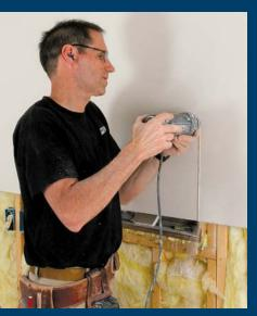
Cut out the sides of the opening with a drywall saw or drywall router.
