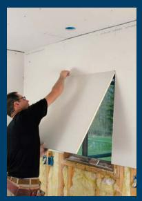
After cutting the sides to the top of the opening, snap the board at the back cut made prior to installation, then finish the cut with a knife.
