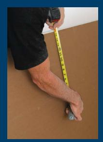
Use the measurements you took previously to score the back of the sheet where the top of the opening will fall, then tack the sheet in place.
