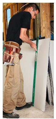
Cut drywall to length using a T-square and a utility knife to score the paper on whichever side is facing you. For the cleanest cut, make one continuous score that goes through the paper face.
