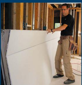
Snap the board, then cut the paper on the other side, starting and ending the cut about 1 in. from the ends to keep the cutoff from dropping. Snap the cutoff forward to free it from the remaining paper. Clean up the edges with a drywall rasp.
