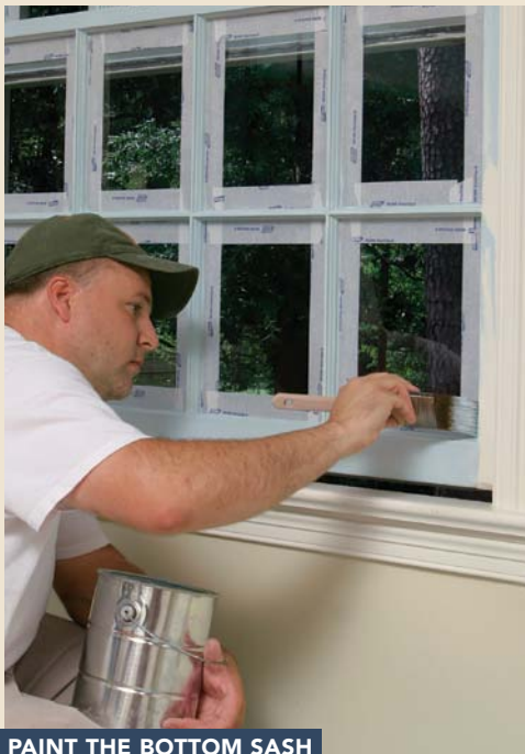
PAINT THE BOTTOM SASH
