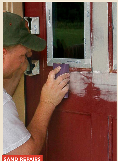
SAND REPAIRS
