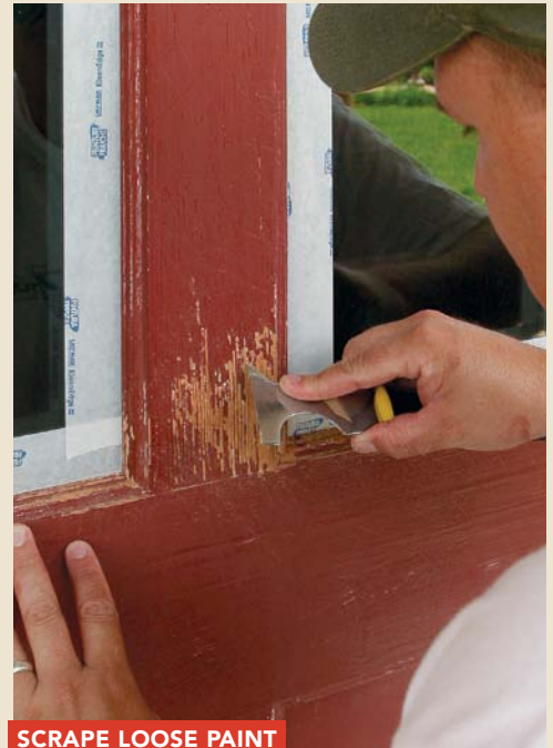
SCRAPE LOOSE PAINT
