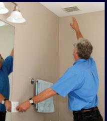
**Don't forget ventilation fans.** Turn off bath fans, clothes dryers, and range hoods before testing. Timer-controlled ventilation equipment such as ERVs and HRVs also should be turned off.
