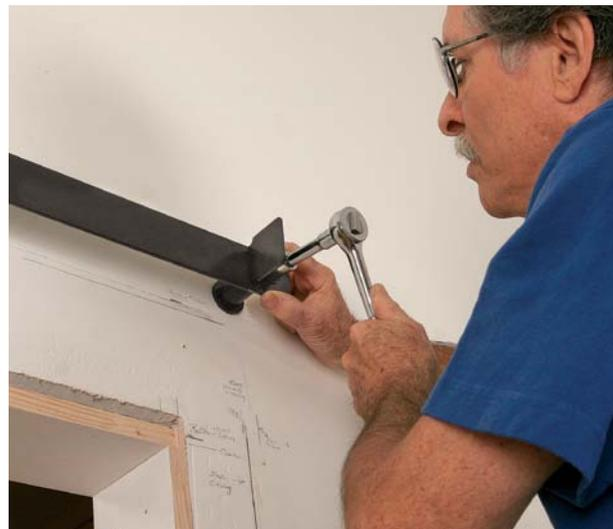
**Fasten the track.** After drilling the holes with a twist bit, fasten the track to the wall with the supplied hardware. Starting at the center, work toward the ends, where the L-shaped wheel stops are located.
