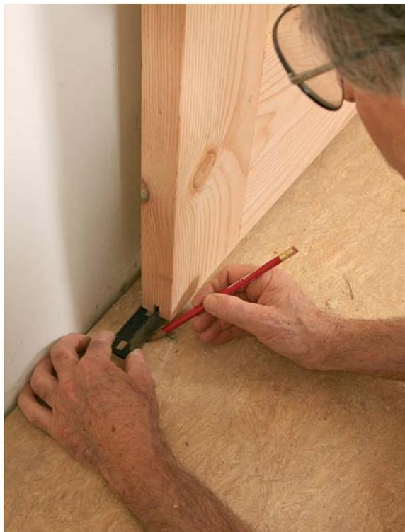
**Mount the guide.** Space the bottom guide from the wall so that it aligns with the track above. One of its two mounting screws is accessible with the door fully open, and the other is accessible when the door is fully closed. This ensures that the door can be removed in the future.
