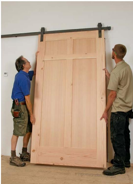
**Hang the door.** Aided by a helper, put the heavy door on the track. Unlike swinging doors, which are partially supported by their jambs, barn doors rely solely on their hardware and its connection to the framing. It's important to correct any weak framing before hanging heavy doors like this one.
