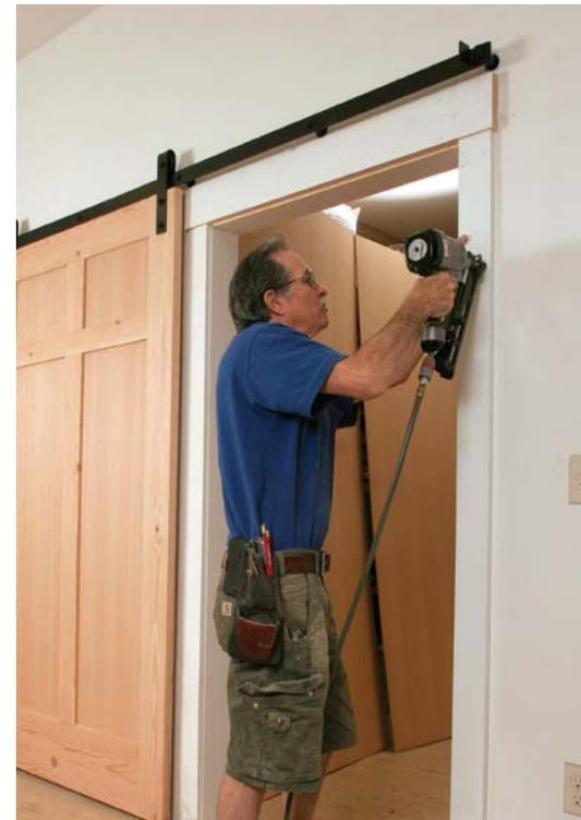
**Finish up with casing.** Barn-style doors are cased like conventional swinging doors. Secure the inside edge of the casing with 18-ga. brads, then fasten the outside edge with 15-ga. finish nails.
