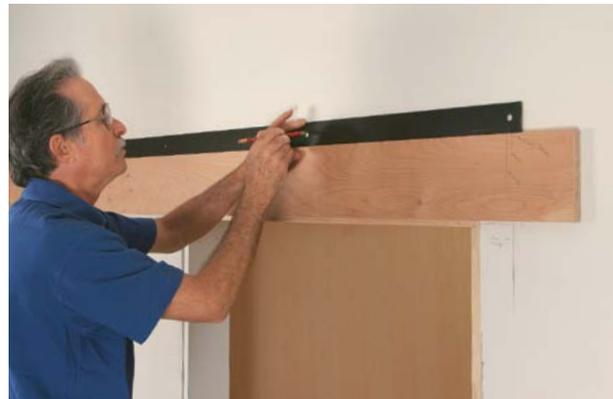
**Mark the holes.** A scrap-plywood ledger holds the track while the screw holes are transferred to the wall. The ledger is the width of the head casing plus 1/4 in. The end is positioned so that it's 1/2 in. beyond the outside edge of the side casing, which accounts for the wheel stop.
