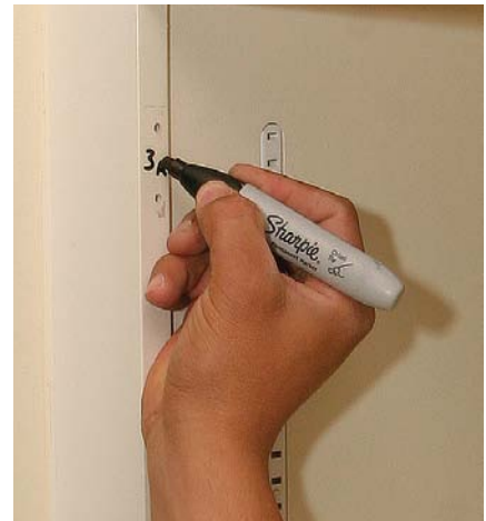
Boxes. Cabinet boxes are marked behind a hinge mount. The void in the finish will be hidden by the hinge.
