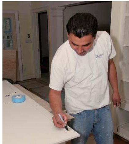
Doors. Cabinet doors are marked behind a cup hinge. The mark indicates which cabinet box the door came from.
