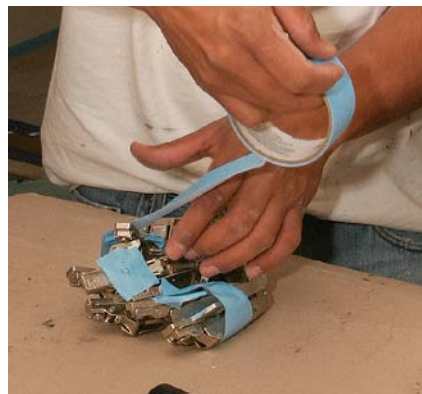
Hinges. Individually labeled hinges are grouped by cabinet door and taped together. Bundles are labeled, too.
