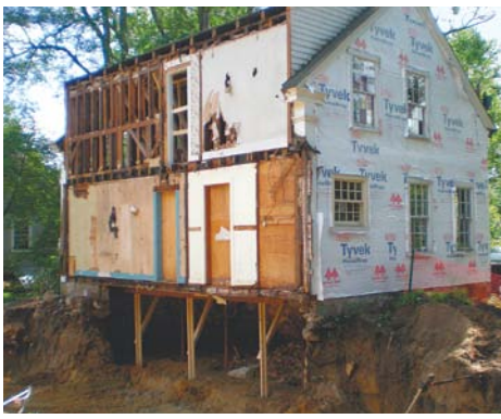
First phase: demolition. After the old additions were peeled away, the main part of the house was supported over the excavated basement in preparation for new construction.
