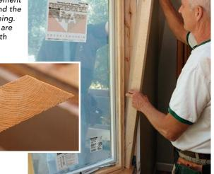
Fasten the sides. With the angled spacers in place, secure the sides of the bay window with 3-in. screws driven through the jamb. The screws are spaced approximately 12 in. apart.
