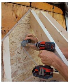
Mount the clamp. The manufacturer provides a paper template for correctly positioning the two-piece cable clamp that anchors the support cables. The clamp location varies depending on the type of bay window used and the blocking or studs behind it.
