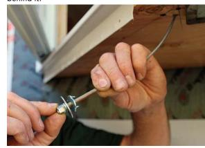
Assemble the cable bottom. The cable's threaded end allows tensioning and future adjustment should the house or window move. The end of the threaded section accepts a hex wrench, so the shaft doesn't turn when the hex nut is adjusted.
