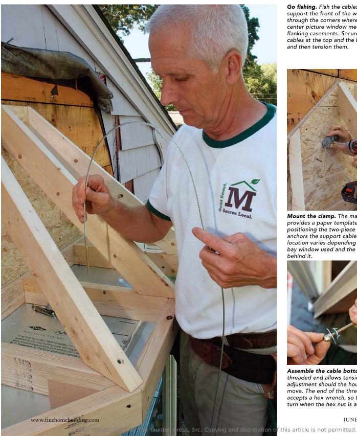
**Go fishing.** Fish the cables that support the front of the window through the corners where the center picture window meets the flanking casements. Secure the cables at the top and the bottom, and then tension them.
