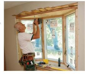
Make angled spacers. A 2x4 with a 45° bevel fills the space between the bay window's angled casement windows and the rough opening. The pieces are best cut with a portable tablesaw.
