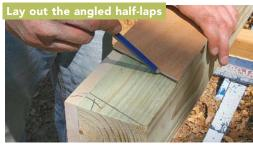
Use the jig shown above to mark the throughcut angle at the top of each rafter, then slide it down to mark the shoulder of the overlap.
