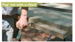
Even with the 71/4-in. circular saw set to its maximum depth of cut, the blade won't be able to finish the half-lap. Use a chisel and a hammer to pop off the waste.
