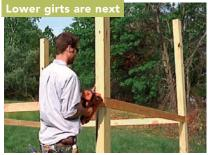
The 2x4 girts, which will later act as the windowsills, provide bracing . between corners and make handy scaffolding for reaching the top plates.
