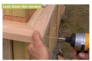
Lock the miters of the sill with a single exterior screw at each corner of the shed. This keeps the miters tight against seasonal movement.
