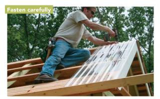
Don't overtighten the fasteners; overtightening can compress their rubber washers and limit panel movement. As with the cedar shingles, use a spacer and ledger to keep the overhang consistent.
