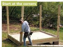
traditional stud wall built on the floor and lifted into place, these walls are built in place, starting with bottom plates and corner posts.
