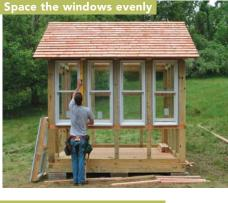
Ripped from 2x stock, 1-in. strips fur out the window opening and provide a nailing surface for the window flanges.
