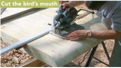
Clamp the rafters together so that the curved ends are flush, and cut the bird's mouth in two passes—first the seat cut, then the plumb cut.
