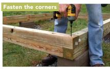
The connections in the frame of this shed are fastened with structural screws. They're available in several lengths and head styles, are weather resistant, and zip into wood without pilot holes.
