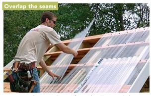
As you work across the roof, overlap the panels by one full trough. The last panel needs to be ripped to width for the proper overhang along the rake. Again, use a circular saw with the blade mounted backward.
