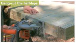
Cut the angle at the top of each rafter, then clamp them together so that their angled ends are in line. After cutting the sides of the halflap with a circular saw, cut across the end grain.
