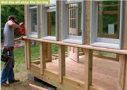
A continuous sill ripped and beveled from 2x stock rests on top of the furring strips, dividing the upper and lower siding and acting as a sill for the windows. Nails are driven through the top of the sill into the furring and the posts for a solid connection.
