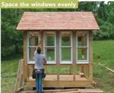
When placing multiple windows with trim in between, leave nice, even spaces between the windows so that you don't have to make tapered rip cuts to fit the trim. Establish the gap between the middle windows. then work to the outside.
