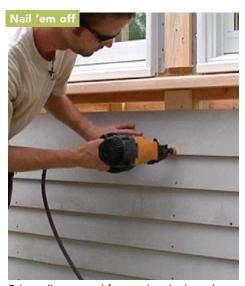
Prime all cuts, and fasten the clapboards with a single siding nail at each framing member. The top clapboard is ripped to 4 in. for an even exposure.
