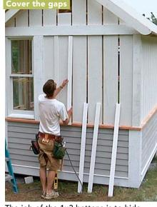
The job of the 1x3 battens is to hide the expansion gaps between the boards and to prevent the boards from cupping. Siding nails should go through the middle of the battens and into the framing.
