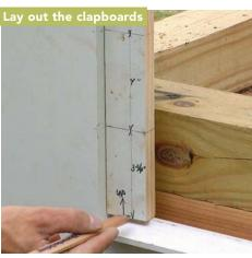
The best way to keep siding in line from one side of the building to the next is to measure and mark the siding exposure on a story stick, then to use the stick to mark the siding exposure on the inside edges of each corner board. Make sure to account for the lip on the back of the drip cap when marking the height of the first course.
