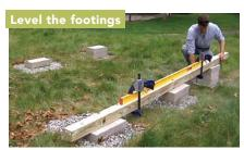
Using the highest corner as a benchmark, level the other corners with the help of a long board and a box-beam level. For fine adjustments, add or remove gravel from the pad.
