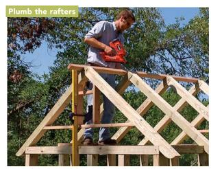
After marking the overhangs and rafter layout on a piece of skip sheathing, nail it to one of the gable rafters a few inches down from the ridge. Next, clamp a level to the framing and tweak this first rafter into plumb. Work your way down the roof, aligning and nailing the rafters to the marked skip sheathing.
