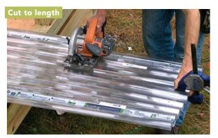
Clamp the corrugated roofing panels together, and cut them to length with a circular saw. To get clean cuts, the roofing manufacturer recommends mounting the sawblade backward. Cutting this material is very loud, so wear ear protection.
