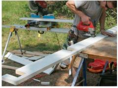
When fitting the fascia board around the rafter tails on the back of the shed, locate the notches by cutting the fascia board a little long, tacking it in place, and using a square and a pencil to mark the cuts right off the rafters. Once it's marked, pull the board back down and cut it with a jigsaw.
