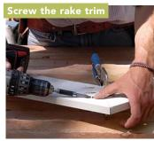
The rake trim will be the outermost part of the roofline, so use pocket screws on the back of the trim to pull the two halves of the miter together and to ensure they never open.
