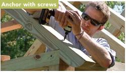
After aligning the rafters to their layout marks, drive a single structural screw through each rafter's bird's mouth and into the top plate.
