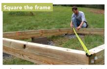
Before fastening the corners of the frame, take diagonal measurements to check for square. They should be within 1/8 in. of each other. If not, persuade the frame a bit with a hammer and a block.
