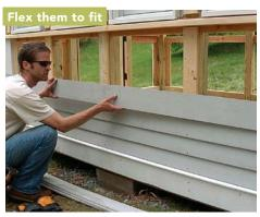
Cut the clapboards just a hair longer than the space between the corner boards so that you can spring them into place for a snug fit.
