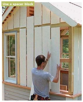
A spacer keeps the board layout consistent. A horizontal trim board will span above the door and windows, making it possible to use short boards on the gable.
