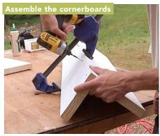
Join the mitered edges of the corner boards with trim screws. Butt the assembly tight to the underside of the sill, and fasten it with ring-shank nails.
