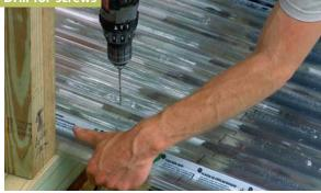
While they're still stacked, mark the sheathing locations on the panels, and drill ¼-in.-dia. pilot holes for the gasketed screws. Drill through the raised portion of the panels, not through the troughs, where water is more likely to seep in.
