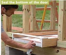
The door doesn't include a threshold because sealing against drafts isn't necessary and having no sill makes the shed easier to sweep out. Without a threshold, though, the bottom of the jamb legs and the door slab must be sealed with primer.
