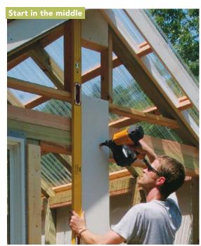
For the board-and-batten siding on the gable ends, start with the center board and work your way out. Make sure to get the first board dead plumb. If it's not perfect, you'll fight the layout all the way across the wall.
