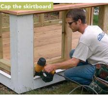
A wooden drip cap is fastened atop the skirtboard, helping to direct water from the trim and spacing out the bottom edge of the first course of clapboards.
