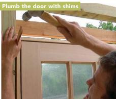
The solid-fir 9-lite door was fitted with a jamb kit prior to installation. Shims at the upper corners lock the door into position temporarily while allowing it to be adjusted for plumb.
