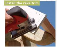
Nail the rake trim to the blocking and skip sheathing, keeping it flush with the top of the skip sheathing. Finish the lower ends of the rake with the same curve as the rafter tails.
