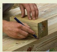
Follow the line, then hog out the waste. The first two cuts establish the shoulders of the notch, and the rest of the passes kerf the lumber so that it can be removed easily. Aim for no more than 1/4 in. between cuts.
