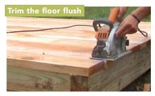
Install the floorboards tight to one edge of the floor frame, then trim any overhang on the opposite end with a circular saw.
