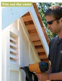
The last step is to install the gable vents, which slide into place from inside the shed and get screwed to the frame. On the exterior, trim above and below the vents ties them into the battens for a clean look.
