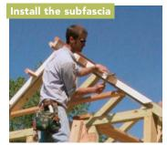
Fasten the rake-subfascia assembly over the furring strips, making sure the bottom of the subfascia lines up with the top of the 5/4 fascia trim that comes later (see drawing above).
