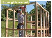
The girt above the door goes in next, but leave the lower girt across the door opening to brace the walls. It can be removed later.
