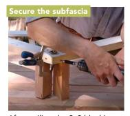
After nailing the 2x3 blocking to each half of the rake subfascia, clamp the halves together at the peak, and drive a couple of exterior screws through the miter to hold it tight.
