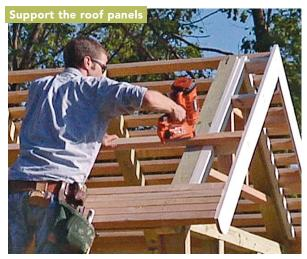
Polycarbonate panels don't need much support, so this side of the roof requires only two pieces of skip sheathing. Align them with the blocking in the fly rafters to help support the fly-rafter assemblies.
