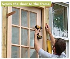
The door jamb must be set out from the frame in line with the ¾-in. furring strips that will back up the door trim. Once in position, the prehung unit is fastened to the frame with screws through both jamb sides.
