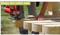
After roughing out the shape of the curve on each rafter tail with a jigsaw, clamp them all together, and clean them up with a belt sander.
