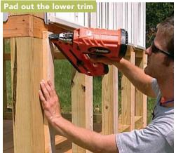
Furring strips are used to space the trim and siding on the lower half of the shed so that they're in the same plane as the board-and-batten siding on the upper half of the shed.
