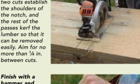
hammer and chisel. Remove the bulk of the waste with a hammer. Then clean up the notches with a wide chisel, leaving the joints reasonably flat and free of high spots.
