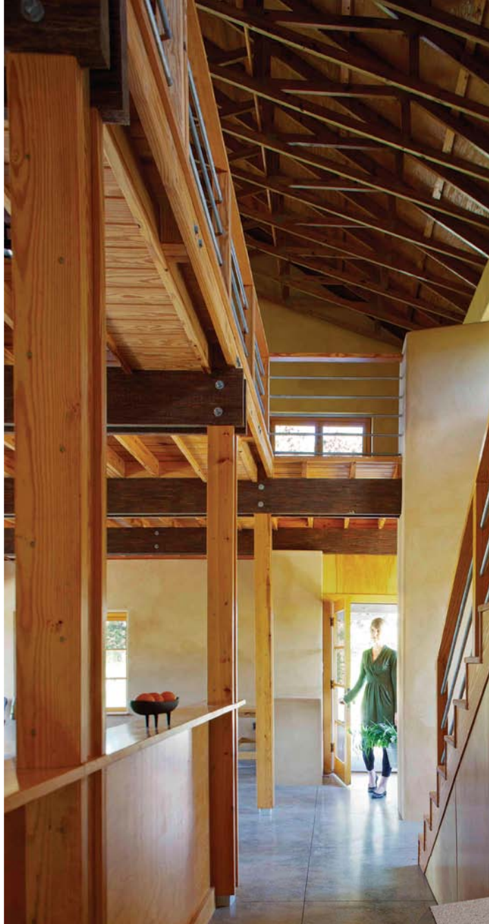
Structure as decor. Just inside the front door, the ceiling opens up to reveal the parade of trusses that support the roof. Throughout the house, its parts are also the finish, assembled with a precision appropriate to trimwork (note the staggered nail pattern in the column on the left). Below, a model enables Govan to get a three-dimensional sense of how the spaces relate to one another in a house. For this one, she used ¾-in.-thick Homasote for the exterior walls.
