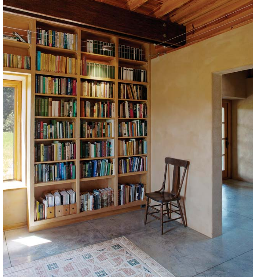
You can see all the parts. In the library, even the low-voltage cables that power the lights over the bookcases are visible. The polished concrete floor is warmed by water from an on-demand heater under the stairs. The mosaic contains patterns from an ancient Roman villa re-created in stone tesserae.
