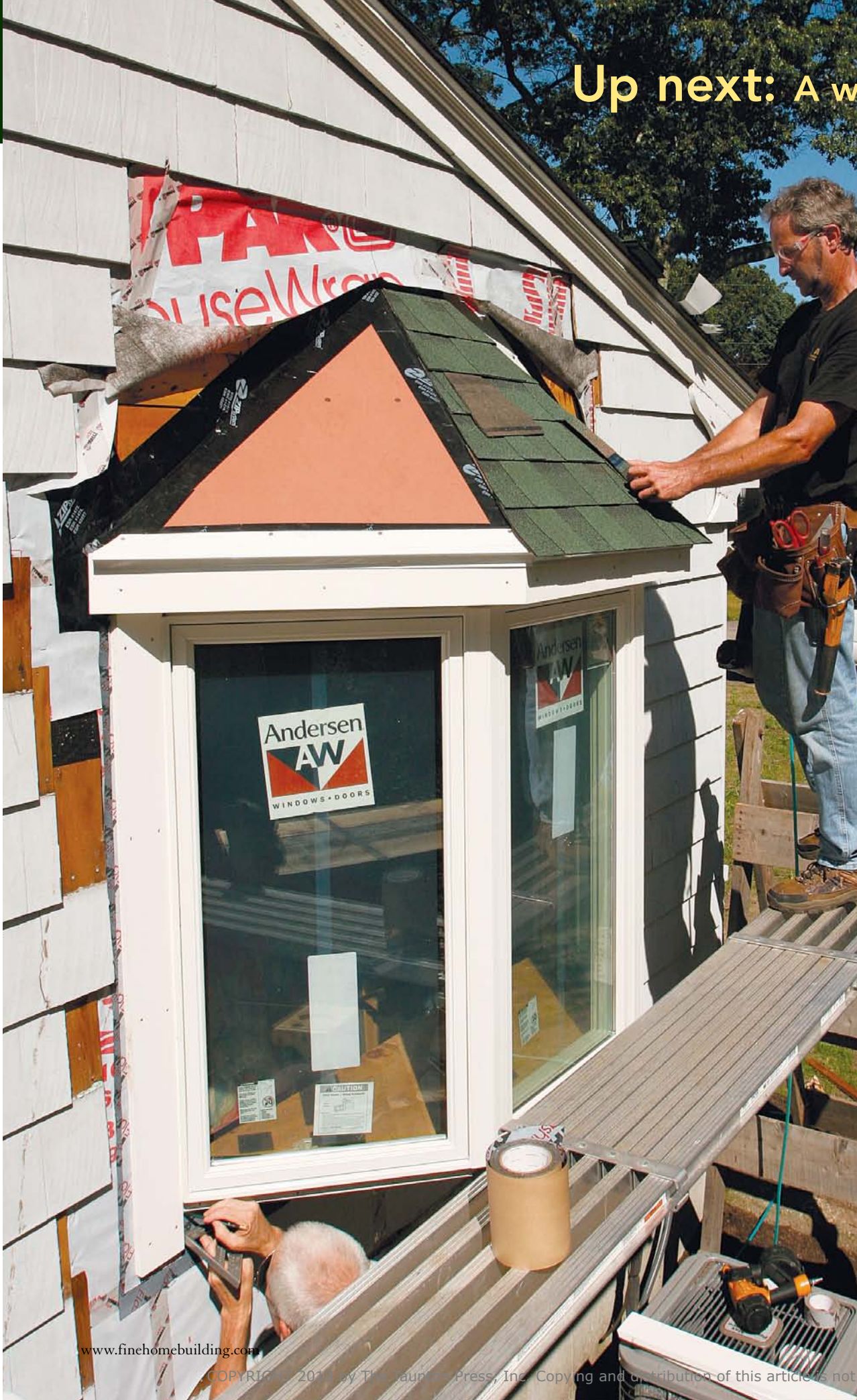
Shimming and fastening
