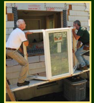
Installing the window
