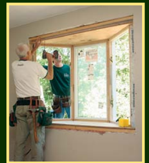
Shimming and fastening
