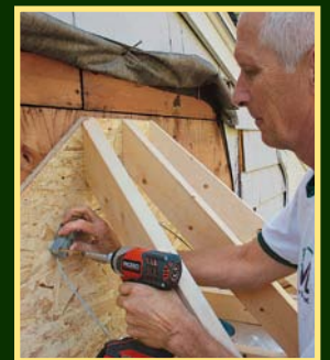
Fastening cable supports
