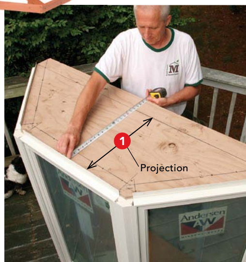
Measure the width and projection. Begin making a template for laying out the ceiling joist and subfascia by copying the shape of the window onto a sheet of 3/4-in. OSB. 1 When making the template, don't include the 4 in. of plywood that extends into the rough opening.
