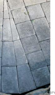
I score at least halfway through each paver when making crosscuts and then split the rest of the way through with a brick chisel. On thin cuts or taper cuts that wedge to a point, I cut the full thickness of the paver. This often means cutting from both the face and the back side to reach all the way through. Small corner nips or edge chips can be made with a mason's hammer.
