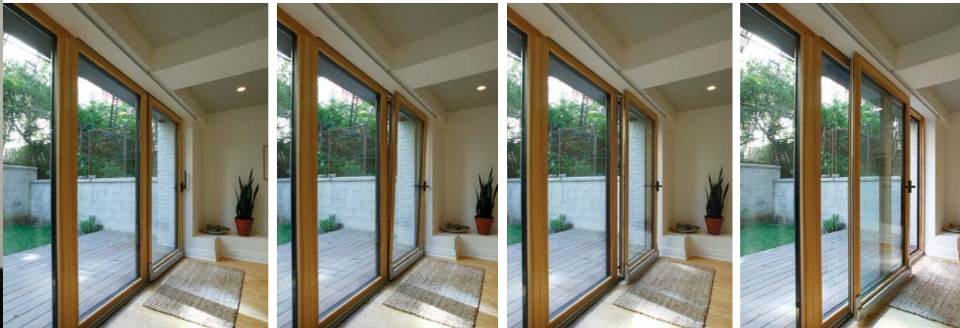
Compression-fit sliders. In the rear of the house, Passive House-certified tilt-open sliders from Bieber connect the interior to the small backyard without compromising the envelope or the historic facade.
