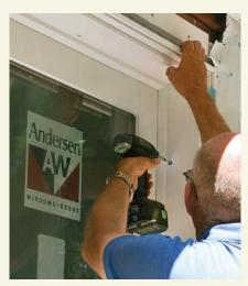
Fasten the door. Once the door is shimmed and square, install the jamb screws, and move inside to check the door's operation. Both panels should latch and lock easily. If necessary, use Pump Wedges to hold the door so you can remove the screws for adjustments.
