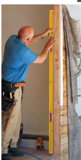
Check for plumb and level. Use a 6-ft. level to check the door opening for plumb and the rough sill for level. It's bet-ter to adjust the door within the opening for out-of-plumb conditions, but correct out-oflevel rough sills with shims or new framing before installing the door.
