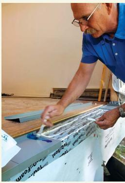
Assemble the pan. This PVC sill pan is shipped in three parts and is field-assembled to match the width of the opening. The sections are joined with PVC cement included with the kit. Between the pan and flexible flashing are three beads of window-and-door sealant meant to keep water and air from blowing under the pan and into the house.
