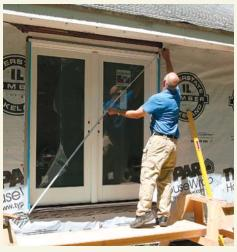
Check diagonals. With two operating panels, French doors are more susceptible to racking than other styles of patio doors. Unequal diagonal meaurements indicate the door is not square and won't operate correctly. If necessary, shim a top corner and recheck until the measurements are equal.
