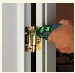
**Strengthen the hinges.** Once the door works properly and the frame is fully fastened, use the 3-in. screws provided to fasten the hinges to the jack studs. This step is necessary to get the door's advertised design pressure (DP) or performance-grade (PG) rating.
