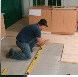
Work from the end. With the position of the sink's overhead light as a starting point, use the kitchen designer's measured drawings to determine the end of the island. Measure from the wall cabinets to create a parallel line that the island will follow.
