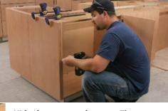
Hide the seams and screws. The seam at the end of the island where the two cabinets meet is often hidden with a wine rack, bookshelves, or panels. This island has a pair of panels that mimic the cabinet doors. The seam between panels is offset from the cabinet seam, locking the cabinets together. Screws installed from the back side are hidden from view.
