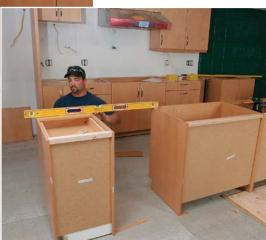
Check across the gap. Where there's a gap in the island's cabinet run for a dishwasher or other appliance, use a long level to ensure that both cabinets are at the same height. Check front and back to confirm that the cabinet tops are in the same plane. Also, make sure that the cabinets are spread the proper distance and that their sides are parallel.
