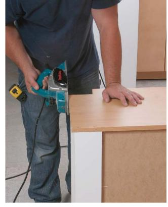
Adjust the height. A few strokes with a power plane quickly remove enough stock to level the cabinet. This planer can remove about ½2 in. with each pass while providing a smooth finish. Deeper passes leave a rough surface. Planing should be limited to a maximum of about ¾ in.
