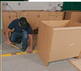
Find middle ground. Many installers find the highest point of the floor to reference cabinet height, and then shim up the cabinets that sit on low spots. A better option is to find a cabinet at average height and then shim the low cabinets up and plane the high cabinets down. Shimming and planing should be minimal.
