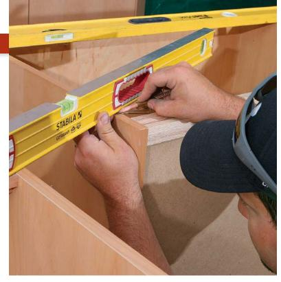
**Lower the high cabinets.** Using a level that spans from a high cabinet to one already at the correct height, center the bubble, and adjust your compass scribes so that they reflect the height difference. Use the same tool to mark the base of the cabinet for planing.
