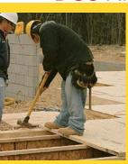
Do use a sledge sparingly. The tongues and grooves on subflooring are designed to gap panels properly, so the panels shouldn't be beaten together except when the tongue has been damaged by rough handling. When that's the case, use a sledge-hammer to get the sheets to meet up. A board prevents the hammer face from doing additional damage.
