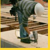
**Do use enough nails.** Nail subfloor panels every 12 in. in the field and every 6 in. along panel edges. Keep fasteners 3/8 in. from panel edges for maximum hold. For 3/4-in.-thick sheets, use 8d (21/2 in.) common nails or gun nails approved by local code. The author uses ringshank nails and adds screws once the house is dried in.
