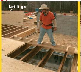
Drop the panel onto the joists as close to its final position as possible; otherwise, you'll mess up the subfloor adhesive when you slide the panel into place. It doesn't matter whether you drop the tongue or the groove edge.
