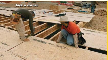
One carpenter moves the sheet so that its leading edge is lined up with the adjacent sheet. Then the nail-gun operator tacks the corner with a single nail. He pauses while his teammate moves the other end into position.
