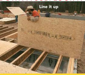
Line up the edge of one sheet with the previous sheet, making sure that all the tongues and all the grooves are facing the same direction. (The author's crew starts with a tongue toward the outside wall.) Don't drag the panels through the adhesive.
