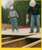
Don't mess up the glue. To prevent smearing the subfloor adhesive, stand the sheet on edge in the proper spot, and let it drop into the glue. A well-timed pull with the ball of your foot can help to keep the panel edge close to the previous row.
