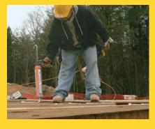
Don't let the glue dry. Apply only as much glue as can be covered with sheathing quickly. Save time by cutting the plastic nozzles on the glue tubes all at once. (An inner seal keeps the opened tubes from drying.) Water-based adhesives, which are more environmentally friendly, work better than they used to, but solvent-based adhesives are still more forgiving in wet weather.
