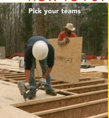
Two carpenters move panels and make cuts while two position, glue, and nail the sheets. While one sheet is being nailed, another is dragged into place.
