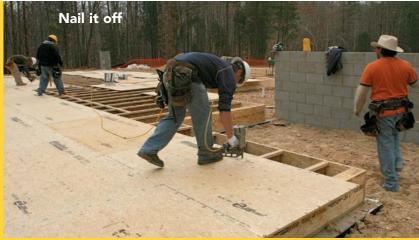
With the sheet in position, the nail-gun operator drives a nail or two to lock the sheet in its final position and then nails the rest of the sheet. With an experienced team, positioning and tacking take seconds. Panels overhanging the edge of the band joist will be cut in place later.
