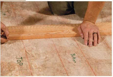
**Reconcile the layout.** After numbering each board's position on the grid, check the accuracy of the marks against those on the floor, and assign the orientation of each dado—whether it will face up or down. Once the horizontals have been marked, check the vertical boards, and mark them in the opposite orientation.
