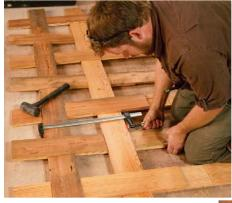
**Pull the weave together.** Run all the horizontal boards from the first vertical, then work in the next vertical. Bar clamps, and later the hammer, help to overcome the resistance of the weave, especially toward the end as the tension increases.
