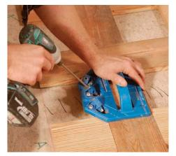
Fasten the grid to the subfloor. The author used a decking jig to locate concealed pocket screws in the board edges. He fastened perimeter ends with two surface-mounted holes that were then plugged.
