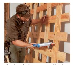
**Glue the underside.** Once assembled, the grid can be moved as a unit. Apply construction adhesive to the back sides of the grid members, then lay the grid back down into place.
