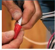
**Neutrals next.** After trimming back <sup>3</sup>/<sub>4</sub> in. of insulation on each wire, join the neutral conductors with a twist-on connector, and fold them into the box.
