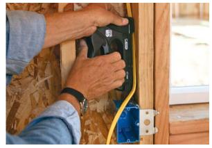
**No loose cables.** The NEC states that cable must be supported horizontally every  $4^{1}/2$  ft. Insulated staples, plastic clips, and drilled holes provide the bulk of the support. Cable must also be supported within 9 in. of a box without clamps, or within 12 in. of a box that has clamps.
