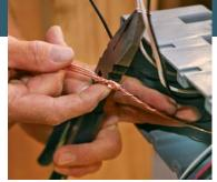
**All grounded.** Twist together the grounds, and secure them with a copper crimp sleeve so there's enough length for each to be connected to its switch.
