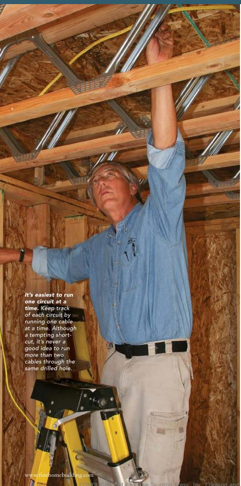
To run cable, feed it up into the joists and to the panel. Leave enough to reach the bottom of the panel, and work back, stapling the cable along its path. Back at the box, estimate about a foot of length beyond the box, cut it from the coil, and then feed the cable through the hole on the top plates and down the stud to the box.
