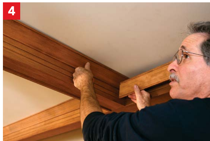
4 Slip it past. Pull out the loose end of the first piece, set the fourth piece in place, squeeze the first piece's coped end over the fourth, and fasten.
