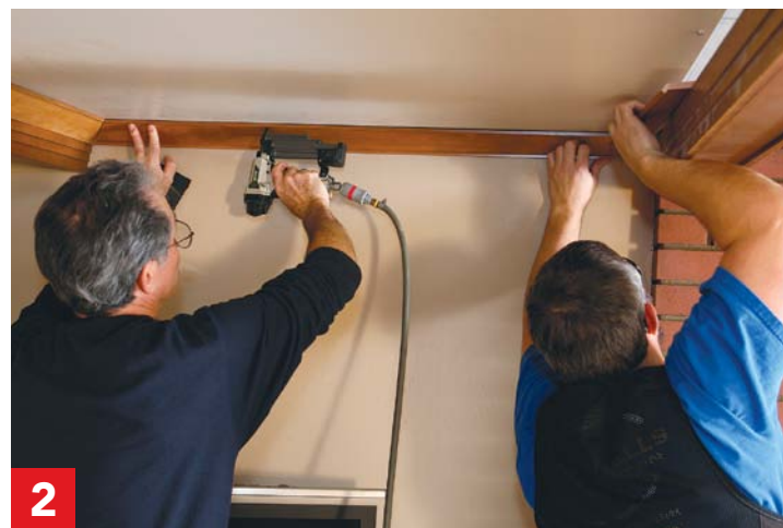
2 Repeat on the second piece. Register the left-hand cope against the first piece, set the angle of the right-hand side, and nail in place.
