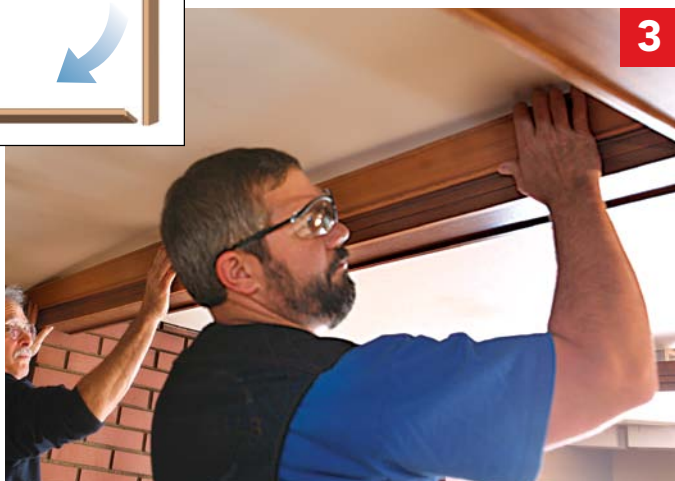
3 Go for a tight fit. When cutting crown to length, be sure to leave the piece a little long so that the cope sits snugly.
