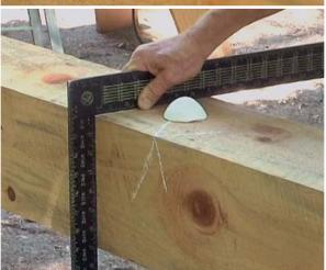
Find the arris. With the timber level, use a framing square to find the two sides that are square to each other. These sides become the reference used for layout, and their intersection is known as the arris. It's a good idea to indicate the arris with a chalk mark.
