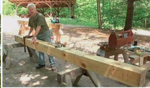
Aim low. The larger dimensions of the timbers create the potential for a higher-than-normal worksurface. Bring down the surface to a normal height by using shorter sawhorses. A 24-in. to 30-in. height is common.
