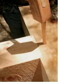
**Lock the joint.** After fully reseating the tenon, drive a tapered drawbore peg into the hole, which draws together the joint.
