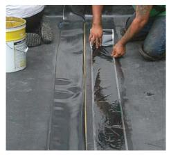
**3** Lay in the tape. The seam tape is placed on the factory-primed lower layer of EPDM with the release paper facing up. Marks made earlier with a white crayon ensure that the seam tape is in the proper position (1/8 in. to 1/4 in. beyond the overlap).
