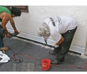
**3** Counterflashing comes next. Above the termination, the crew installs a shop-formed, 0.040-in.-thick, white aluminum length of nail-on counterflashing. The counterflashing is installed similar to the termination bar. A continuous bead of water-block mastic is placed behind the flashing, and urethane sealant is spread on fasteners and along the top edge.
