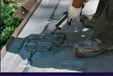
Lap cement seals tape edges. Once the membrane and flashing installations are complete, both sides of the flashing tape and any overlapping membrane should be wiped clean with weathered membrane cleaner and sealed with EPDM lap caulk.
