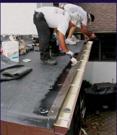
Nail, then prime. Edge metal is set in a bead of water-block mastic. Once the edge metal is in place, fasten it with 1½-in. galvanized roofing nails arranged in a staggered pattern every 6 in. on center. The edge metal and the adjoining EPDM then are wiped with membrane cleaner and primed with EPDM primer.
