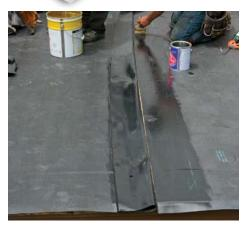
**Prepare seams with primer.** An application of primer boosts the seam tape's adhesion. It's important to apply the primer along the full width of the seam and to both layers of EPDM.
