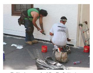
Flashing improves durability. The flashing is attached every 12 in. with expansion anchors. The installation of the nail-on counterflashing effectively doubles the life of the wall termination to 20 years or more, and the painted aluminum looks better than the exposed termination bar.
