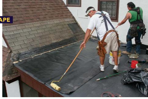
**1** Bridge transitions in roof slope. This transition between the house's low- and steep-slope roofing created ice dams that forced water under the shingles and rotted a section of sheathing. The author solved the problem by covering the transition with the EPDM membrane. Replacement shingles will be installed later.
