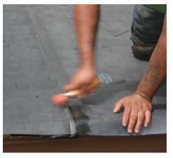
**7** Roll again. The top layer of EPDM then is rolled into the seam tape much like the lower layer. It's important for every bit of seam tape to be rolled thoroughly to activate the pressure-sensitive adhesive.
