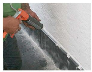
**2** Caulk the termination bar. The bar is installed so that the factory-formed kick sticks out from the wall. The kick is filled, and the fastener heads are coated with high-quality urethane sealant.
