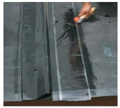
**4** Roll the seam. Every inch of the seam tape is rolled vigorously with a 3-in. neoprene roller. It might be tempting to use a wider tool to save time, but bigger rollers don't exert enough pressure and are not approved by EPDM manufacturers.
