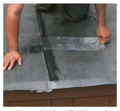
**Remove the release film.** Remove the film by slowly pulling it away from the seam at a 45° to 90° angle. Use your other hand in a sweeping motion to bring the top layer of EPDM over the seam tape.
