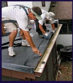
Tape seals the deal. Peel-and-stick cured flashing tape is used to seal the metal edge. The tape keeps the joint watertight despite the inevitable movement that occurs between the edge metal and the adjoining EPDM. It's rolled in to activate the adhesive.
