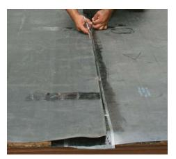
**Trim to fit.** If less than ½ in. of seam tape is showing, the top layer of EPDM should be trimmed. Heavy-duty scissors are the best tool for cutting EPDM membrane.
