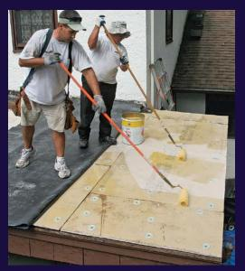
**Spread the adhesive.** EPDM is glued down using a special adhesive similar to contact cement. It's rolled onto both the gypsum sheathing and the back of the EPDM membrane. When the solvents have flashed off (20 min. to 40 min. in warm weather) and the adhesive is tacky, the EPDM is laid in, and the surface is swept with a broom to ensure that it's fully adhered.
