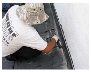
Termination bar is first. The upturned EPDM membrane is coated with bonding adhesive almost to the top. Then the uncoated area receives a continuous bead of water-block mastic. Once the two adhesives are in place, an extruded aluminum termination bar secured every 8 in. with Zamac expansion anchors (www.powers.com) holds the top edge.
