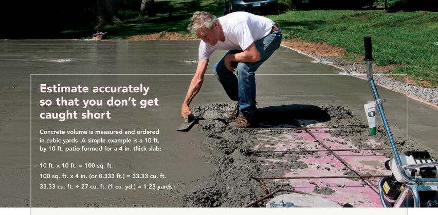
One sure way to create havoc and possibly ruin a job is to come up short on concrete. There are lots of ways to lose concrete: Forms can spread, holes can be overexcavated, chutes can overflow, concrete can be spilled, or there can be a change in volume from loss of air entrainment or settling in a wet mixture. Unless your job site is next to the ready-mix plant, chances are that the short load of concrete you just poured will have set up by the time the makeup
