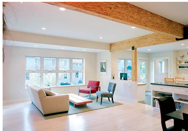
Big beams open the floor plan. To open the first floor, a couple of major bearing walls had to be removed. Rather than wrap them with wood, the owners chose to leave the parallel-strand-lumber beams exposed to give a modernist flair to a traditional detail. Photo taken at D on floor plan.
