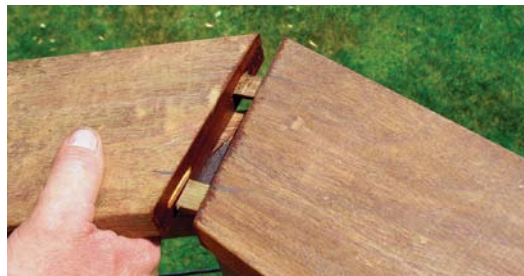
Cap rail ties it all together. You can use 5/4x6 decking or 2x6 stock attached with screws for a top rail. The resulting "T" between the cap rail and the subrail forms a strong top-rail system. Joints can land on top of a post or along a subrail span. Use dowels or biscuits to keep the joints tight and cap-rail pieces in plane with one another.
