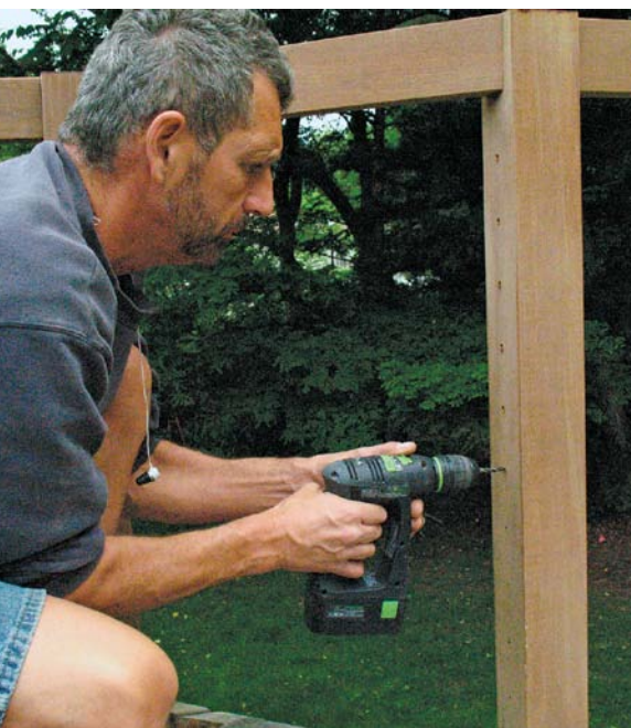
Flash forward. When cable enters or exits a post at an angle, sleeves are needed to protect the wood. Rather than oversizing holes for the sleeves during the production boring process, the author drills out the larger holes after the posts are in place. The cable sleeves require a countersink to accept the flare at the end.
