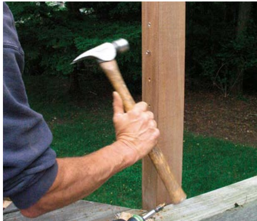
Install cable sleeves. Swipe the holes bored earlier with a piece of sandpaper to clean off any wood fibers and to allow the sleeve to sit nicely in the post. Gently tap the sleeves into position.
