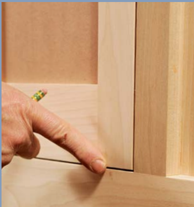
When a door goes wrong. A warped door won't land evenly on the strike side and may protrude beyond the face frame at the top or bottom.
