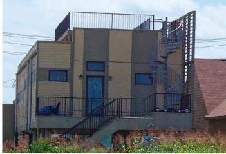
A way out. All MIR homes provide a roof escape in case of flooding—either a hatch (top photo) or a roof deck (bottom photo), which also can be used for recreation.
