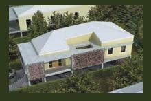
The sloped design by the New Orleans-based firm Concordia (photo above) is intended to maximize solar collection and to promote passive ventilation. Its floor plan, like that of many MIR houses, reinterprets the traditional shotgun layout in which rooms are arrayed one after another.
