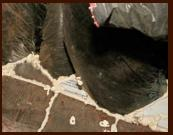
Seal the ceiling or floor. When the joist bays are blocked with pipes or ductwork, seal the floor around them to stop air movement. Here, the author is cutting foam to fit around insulated flexible duct. For maximum benefit, the gaps between floorboards must also be filled with foam.
