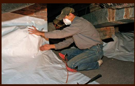
Cover the soil. A heavy-duty reinforced plastic liner is placed on the crawlspace's dirt floor. Seams are covered with special tape, and the plastic is lapped onto the brick piers that support the house. The laps are first glued to the piers with solvent-based construction adhesive and then secured with the seam tape. At one time, the author used troweled mastic for sealing seams, but the tape is neater, is faster, and performs just as well.
