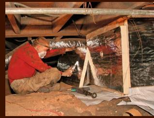
Insulation prevents heat loss. A layer of 1½-in., foil-faced polyisocyanurate is put over the poly sheeting. The insulation is held in place with 2½-in. powder-actuated pins with 2-in. washers. Seams are covered with 2-in. foil tape.
