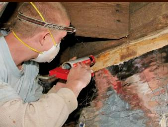
A Separate inside from outside. Built with rigid insulation, pressure-treated lumber, and canned spray foam, walls separate the cold outdoor spaces under a pair of porches from the conditioned crawlspace.
