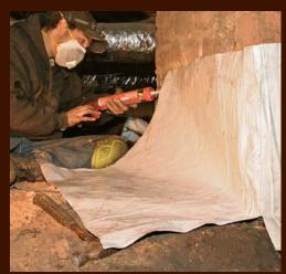
**2** Cover the walls. The foundation walls are covered with 12-mil reinforced poly sheeting to stop the flow of air and moisture into the crawlspace. The poly is held in place with a thick bead of solvent-based construction adhesive.
