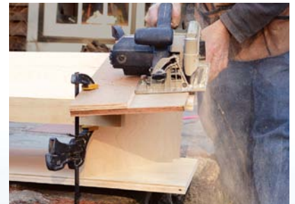
A saw guide is a must. When trimming scribed cuts, a site-built saw guide is a fast way to make an accurate cut.
