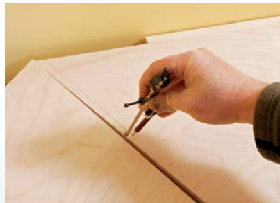
A scribe may be necessary. Position the opposite side base, and check the fit. Use a set of scribes to mark the cut.
