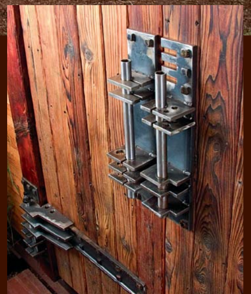
Montgomery designed and fabricated the custom door pulls and hinges.
