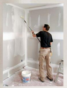
**Get rolling.** Start at a corner and work toward the opposite wall. You can coat about 24 sq. ft. to 30 sq. ft. before the compound starts drying. This room will get wainscoting, so the author isn't skimming the bottom 3 ft. of the wall.
