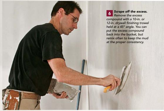
**LEVEL 4** This level has joint tape embedded in compound and two additional coats of compound on top to hide the tape and to smooth the surface. Fasteners are concealed with three coats of compound. Finally, the compound is sanded with fine-grit paper and primed. This level of finish is not recommended under gloss, semigloss, or enamel paints.
