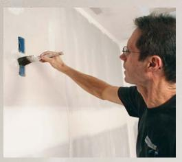
Wipe down the walls. Brush down the walls with a soft push broom, and scrape off any errant blobs of compound that could interfere with skim-coating. A 2-in. paintbrush is great for cleaning out electrical boxes.
