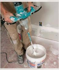
Thin out the mud. Use a heavyduty drill with a paddle to mix up the compound. Add water a little at a time until the mud's consistency is similar to pancake batter.
