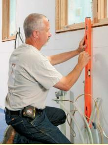
4 Mark cabinet locations. Draw plumb lines on the wall to establish cabinet positions, taking care to be sure that cabinets such as the sink base align perfectly with the windows above.
