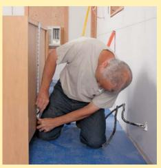
1 Modify for services. Measure the distance from the cabinet layout lines on the wall to the services coming through the wall or floor. Transfer the vertical and horizontal measurements to the back or bottom of the cabinet, and cut a hole with a hole saw that's slightly larger than the size of the service line being accommodated.
