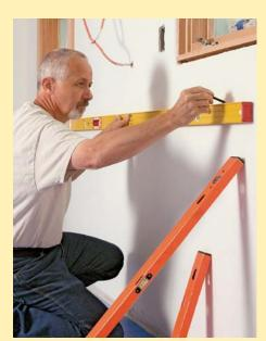
**3 Draw** a **level line** across the wall. Connect the marks on the wall with a level to establish a line to hold the base cabinets to during installation. This technique is more accurate than snapping chalklines or using a laser-level line.
