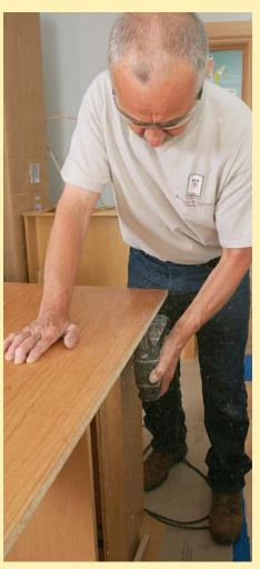
4 Cut the waste. Bulk material can be removed with a track-guided circular saw or a jigsaw. Follow the scribe line closely, but leave the pencil line.
