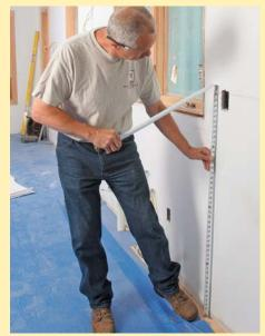
**1 Find the high point in the floor.** Measure the distance between the floor and a laser-level line about 4 ft. above the floor to find the high and low points in the floor. The high point dictates the height of the base cabinets; use shims to compensate for the low points in the floor.
