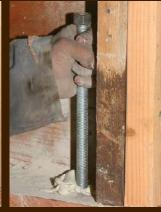
3 Set the rods. After filling the holes with epoxy, set the 5%-in. all-thread rods. Twist the rods to ensure the epoxy finds it way between each thread. The epoxy used is quick setting, and the nut will be ready to tighten within an hour.
