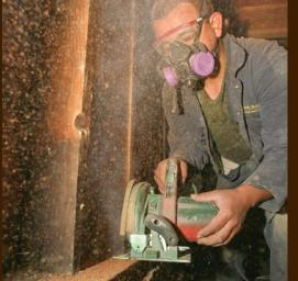
1 Cut the mudsill flush with the studs. This allows the plywood to be edge nailed against an even surface. This is best accomplished with a tool like the Closecut saw by Clemenson Enterprises Inc. This photo shows a saw modified with the FlusSa attachment.
