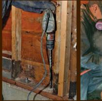
2 Drill and prep holes for hold-downs. With a rotary hammer drill and masonry bit, drill an <sup>11</sup>/<sub>16</sub>-in. hole at least 12 in. deep. To ensure a proper bond between the epoxy and the threaded rods, plunge each hole with a bottle brush, then blow compressed air into the hole to remove masonry dust. Repeat this process three to four times before dispensing epoxy into the hole.
