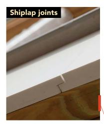
Shiplap joints. When there's an outside miter at both ends of a trim run that's 12 ft. or longer, use two boards connected with a shiplap joint to allow the boards to move without exposing the material underneath the joint.
