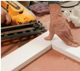
Miter joints can be joined with plastic biscuits. The author coats the biscuit and both sides of the miter with PVC cement, then assembles the joint. The corners can be tacked with a finish nail to hold the joint tight until the cement sets up.
