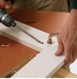
When assembling casings with butt joints, the author prefers to apply PVC cement to each joint and then to draw the joint together with pocket screws.
