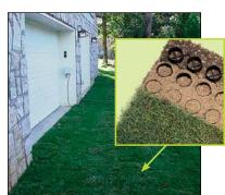
Permeable paving. Impermeable surfaces should be replaced with permeable products that help to keep your lot moist and cool. This driveway is made of Grasspave2 by Invisible Structures Inc.
