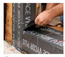
Wrap the sides. Cover each side of the rough opening with flexible flashing. Extend the flashing down over previously applied layers as far as possible. A single slit allows the flashing to be wrapped inside the opening and integrated into the beveled sill.
