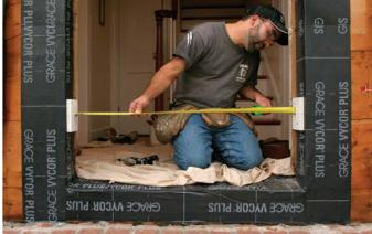
Plumb up. With the distance between the lower screws set, plumb up the side of the opening. Adjust the upper screws so that they are plumb with the bottom screws.
