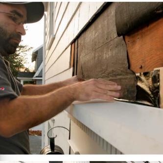
Restore the drainage plane. Starting at the bottom of the door and working toward the top, peel away the paper backing on the back-flashing, and stick the housewrap to it, making sure that each piece is lapped over the piece below it. . The back-flashing, which is sealed to the beveled PVC head casing and is woven into the housewrap, eliminates the need for metal cap-flashing.
