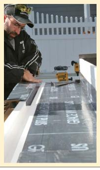
Back-flash the casing. Flexible flashing seals the joint between the jamb and the trim. A strip of flashing with the paper left on the exposed adhesive side should extend 4 in. beyond the trim. The flashing will be woven into the housewrap once the door is installed. A single strip of flashing can accomplish both tasks on narrower trim.
