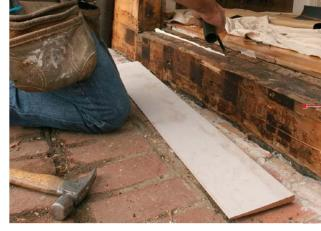
Create a seam-🚄 less base. Held to a plumb line on the sheathing, the first piece of flashing extends across the bottom of the opening. A slit on each end allows the flashing to wrap over the sill and extend up the face of the wall.
