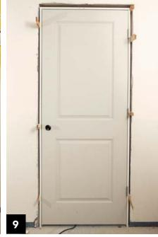
1. Two carpenters are better than one. Alex has a 6-ft. level, and he stands on the interior of the door to establish a plumb hinge side and to check the gap around the door. Tucker stands at the door's exterior with shims and a nail gun. Alex can see when each jamb's gap is consistent and tells Tucker when to adjust or nail.
