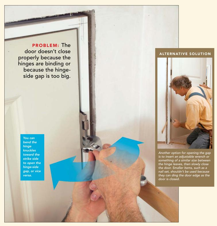
**SOLUTION:** Carefully bend the hinges. If the hinges are binding, the gap is too tight. To open the gap, use a crescent wrench to bend the jamb-side hinge knuckles toward the door handle. To close the gap, bend the knuckles away from the handle.
