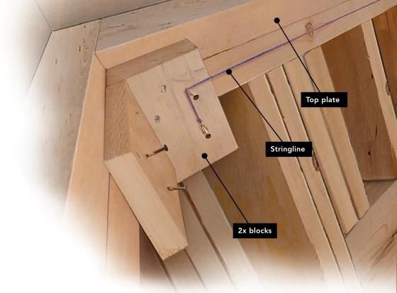
illustration above. These nails act as anchor pegs for the string. Many framers use strong mason's twine for stringing because it can be stretched extremely taut. A chalkline can work just as well, though, and it has the advantage of having a hook on the end that can slip over the bottom nail on one block.
