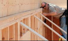
**Double-check the string.** Once all springboards have been adjusted, go back and sight down the stringline to make sure that the wall is straight. Now is the time for any last-minute tweaks, before the top plates are locked into position by the joists above.
